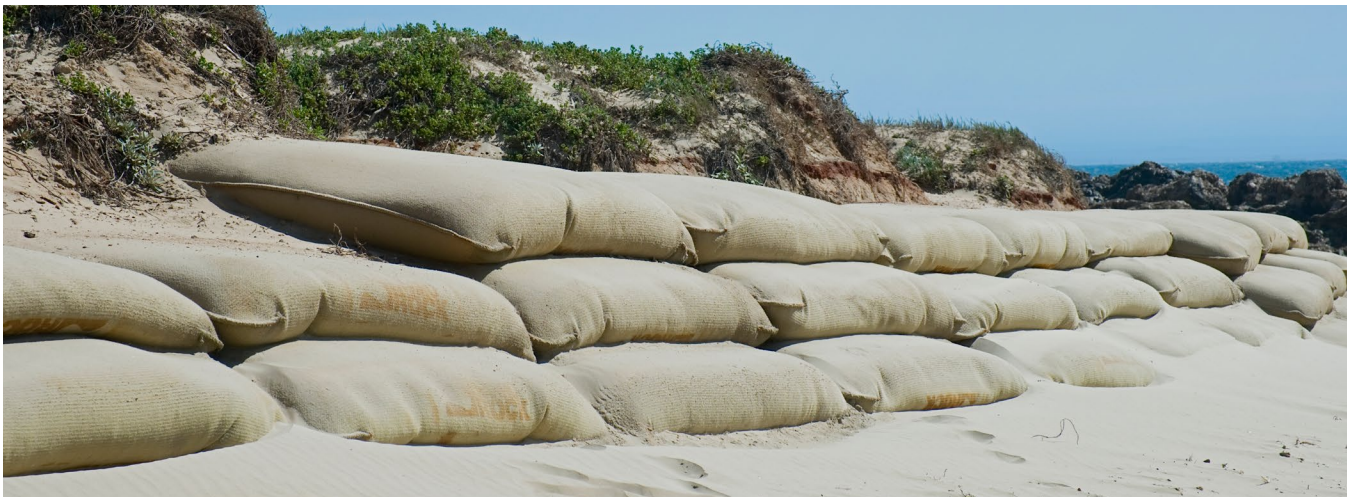
Large sandbags placed on the beach to stop erosion during high tide and stormy conditions. (© Michael Sheehan / Shutterstock)
