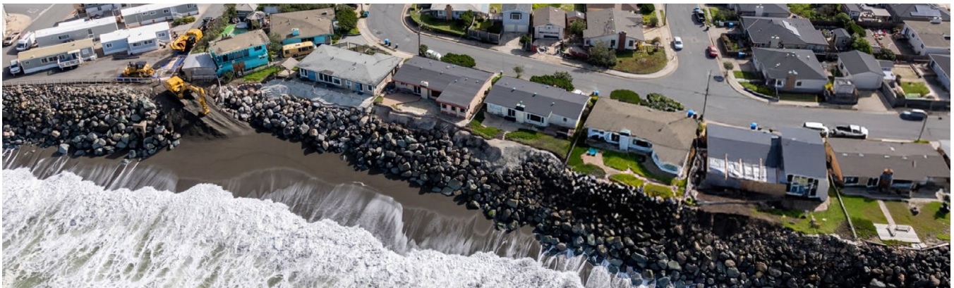
A rock seawall protects homes from erosion in Pacifica, California. (© JasonDoiy / Shutterstock)
