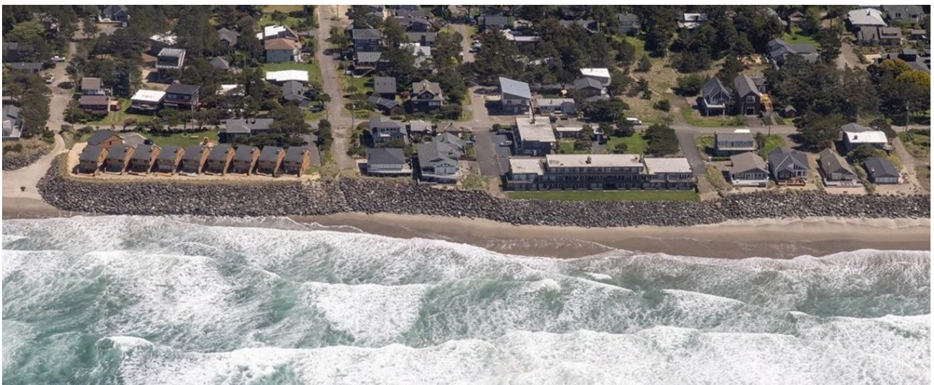
Extensive riprap placed on the beach in Neskowin, Oregon, makes stretches of beach impassable. (© Rena Olson)
