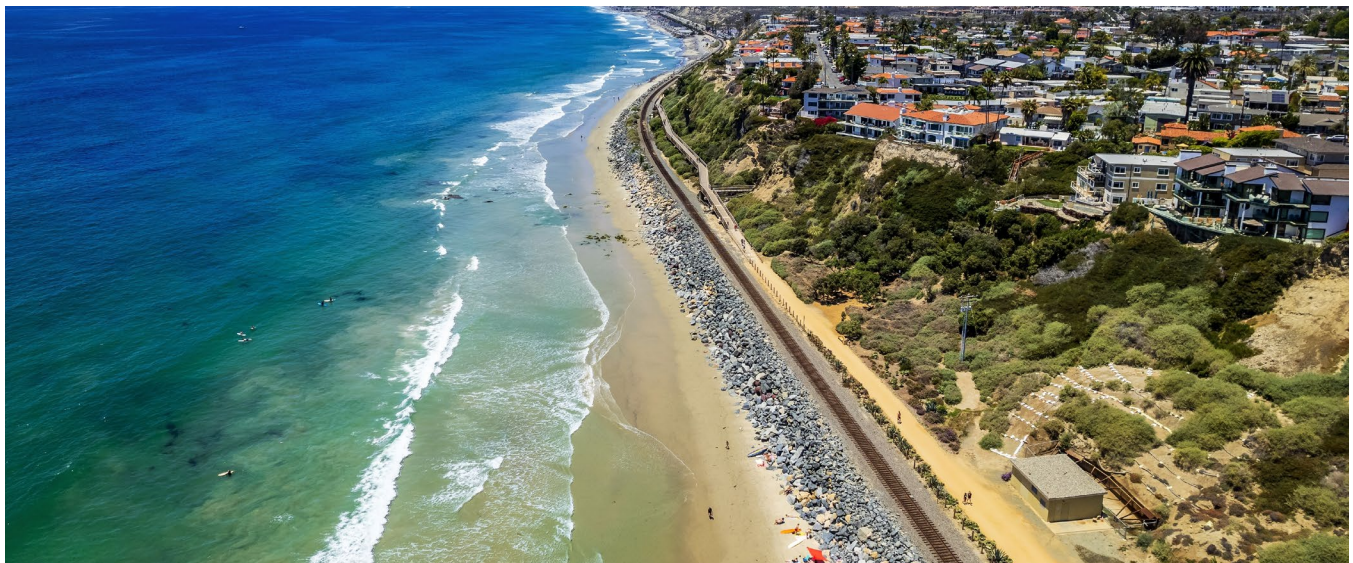
Orange County Transportation Authority's (OCTA) existing rock riprap along the San Clemente coastline. (© CameronCreatives / Shutterstock)
